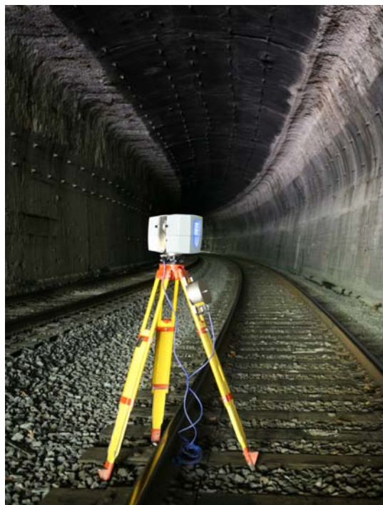
The FARO Laser Scanner preparing for a scan inside the Twin Branch 1 tunnel
